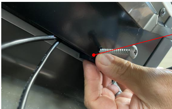
Tuck Wire Connector Under Sash and Install Screw. Ensure Wires are above Screw.
